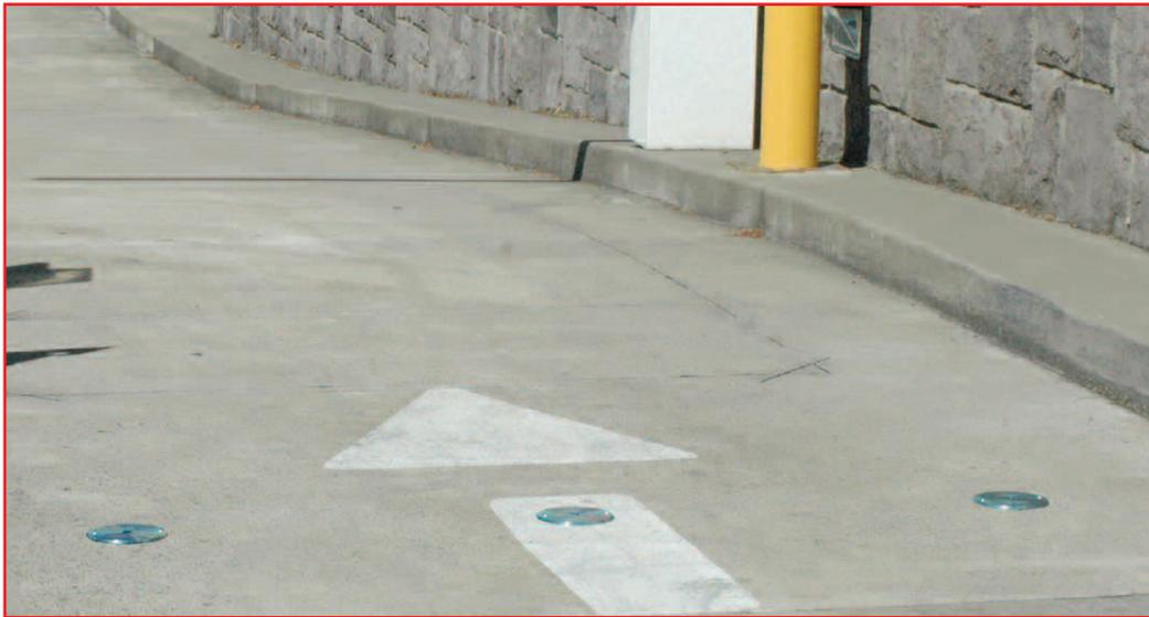
*Like the Mini's taller siblings, the Mini's magnetic base attaches to the plate epoxied to the surface, allowing consistent placement.*
