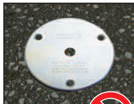
No or Wrong Epoxy
