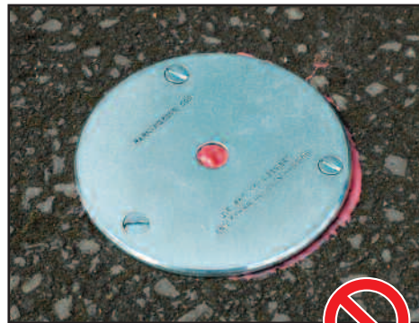
Epoxy in Center Hole
